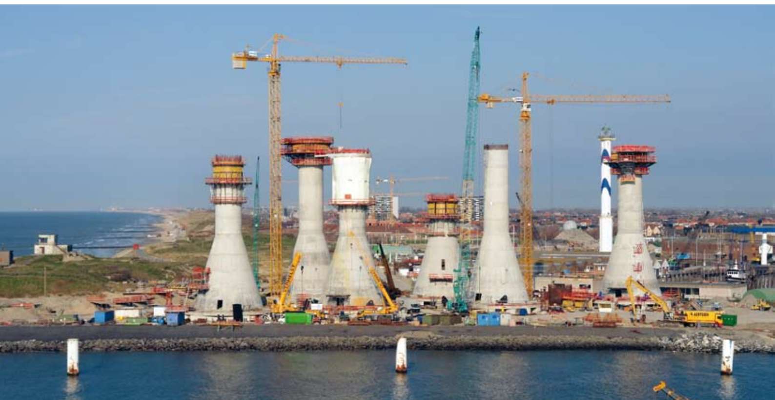
CONSTRUCTION OFFSHORE WIND FARM, BELGIAN COAST
