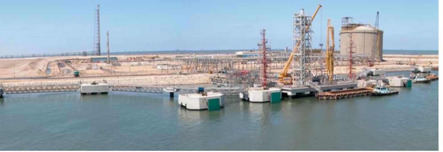
DAMIETTA TERMINAL EXPORT FACILITIES, EGYPT
