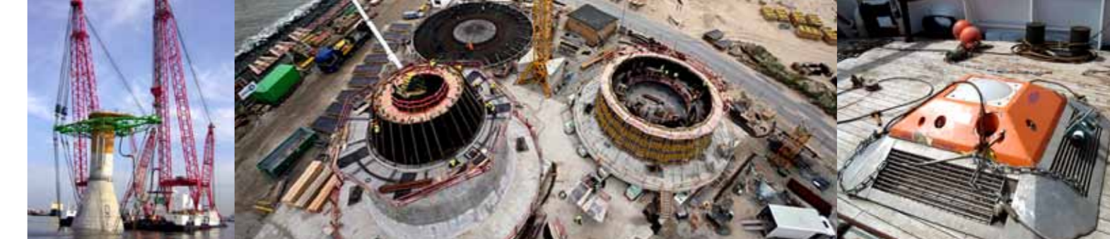
OVERSEA TRANSPORT OF FOUNDATIONS
